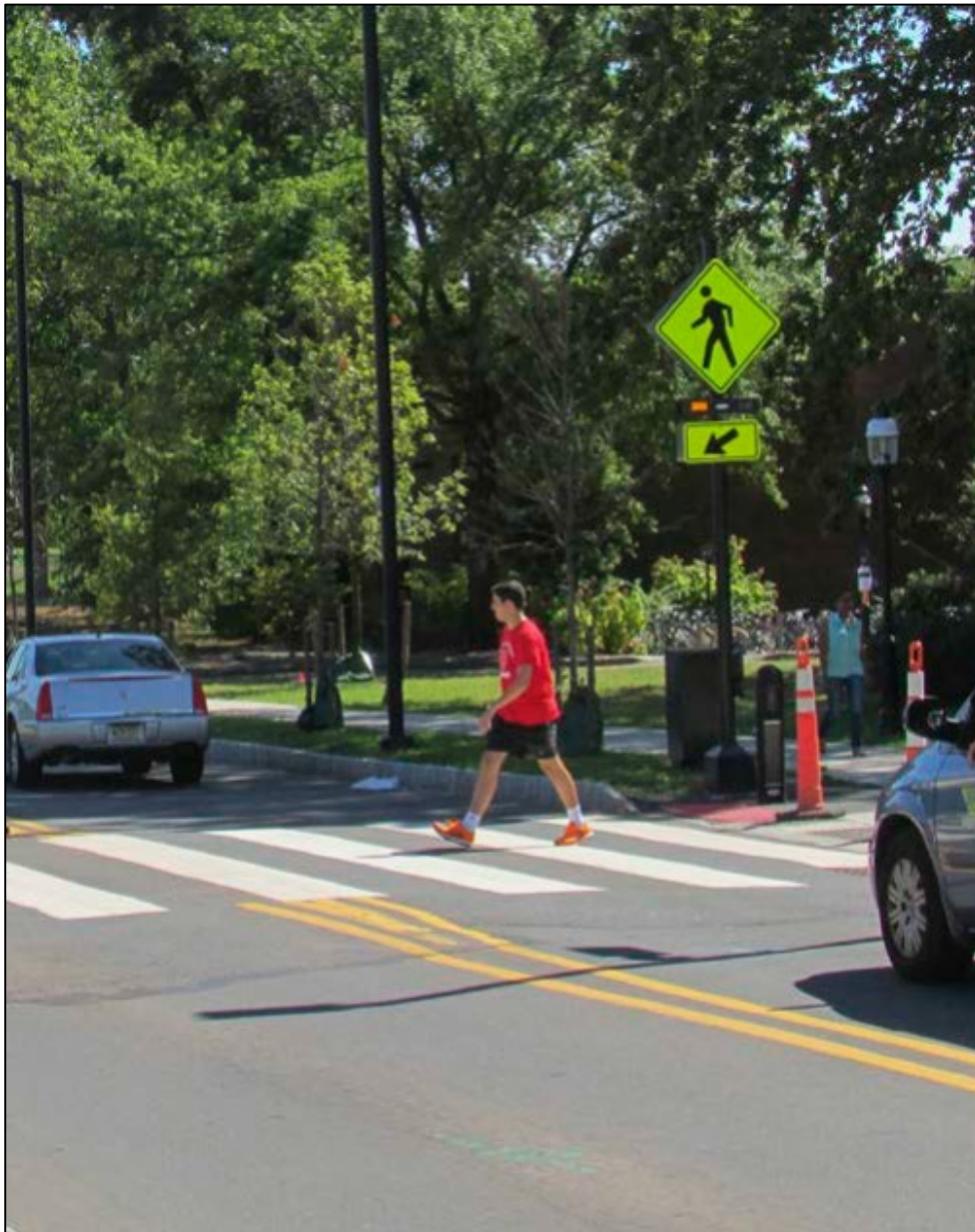
Figure 51: Rectangular Rapid Flashing Beacon (RRFB)
