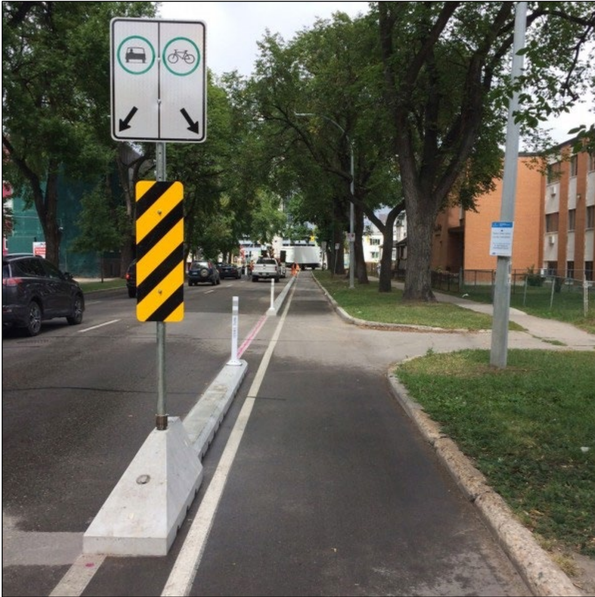
Figure 62: Temporary Concrete Bike Facility in Winnipeg, Canada
