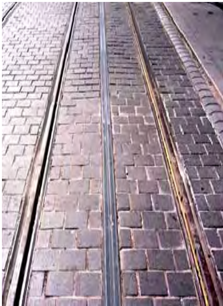
Figure 1-18 Bordeaux tracks with imbedded traction power
